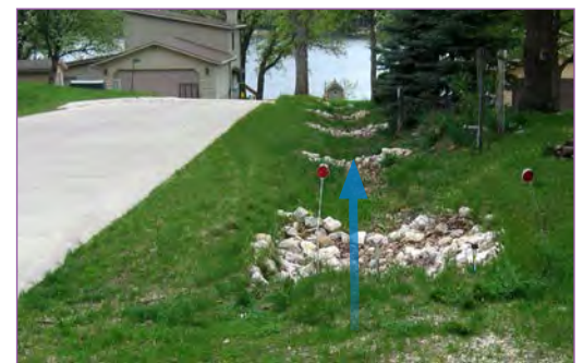
Dickinson County Bioswale
