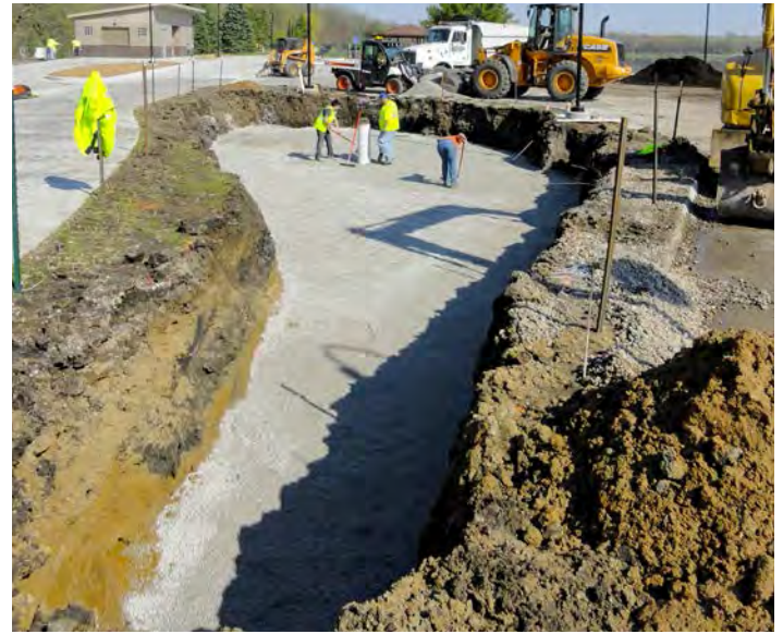
STEP 2 Installation of Rock and Overflow Pipe
