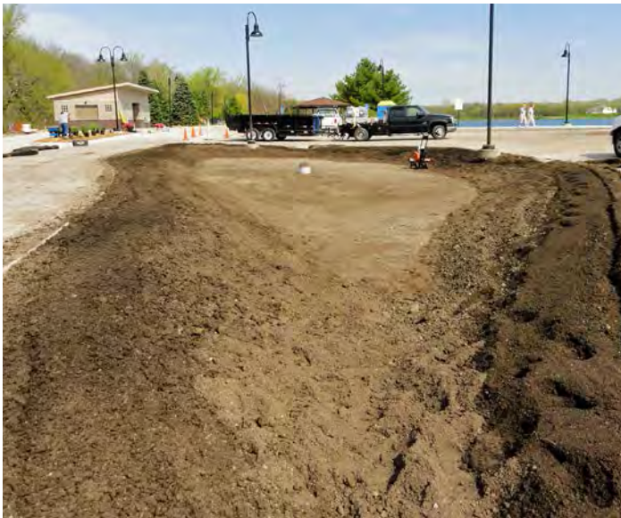
STEP 3 Placing the Soil Media
