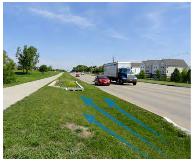
Pre-treatment swale for Ankeny biocell
