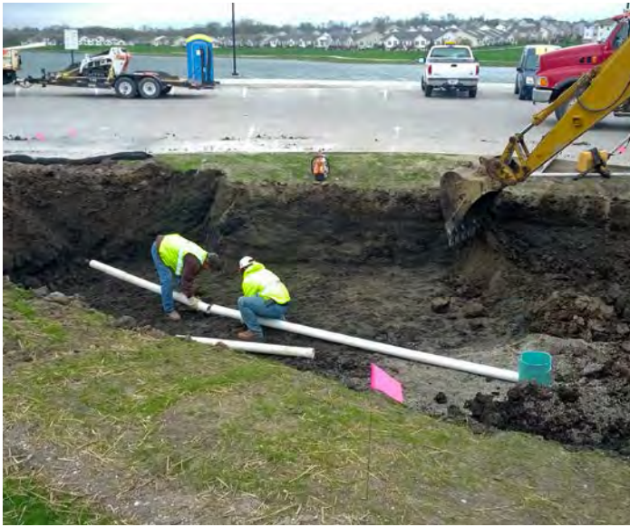
STEP 1 Excavation and Installation of the Subdrain
